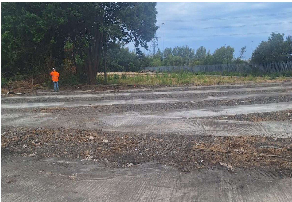
Plate 1: General view of site
