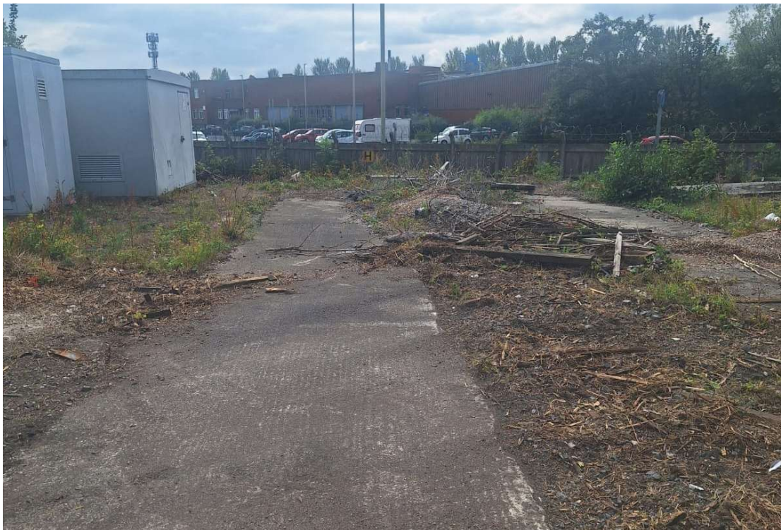
Plate 3: General view of site facing south
